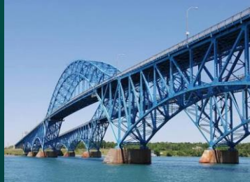
Structure – construct bridges
